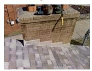
Flashing is usually thin sheets of aluminum or galvanized steel. Many professional roofers will fashion their own from sheet metal. Flashing is installed over joints in the roof & wall construction. Possible areas are valleys, chimneys, dormers, windows, pipes, skylights, porches, decks and edges.
