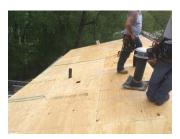
This is the wood that makes the solid structure of the rooftop. During a roof replacement project, it may be discovered that some of this decking has been damaged and needs to be replaced. A roofing contractor may indicate this expense in different ways. If they see obvious damage they will note that in the estimate and the type of material that will be used. This could be plywood, Luan or other coverings. However, sometimes this damage is hidden until
