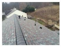
most popular are ridge vents. They are installed along the ridge or peak of the roof and allow hot air to escape and draw cool air in the soffit vents.
